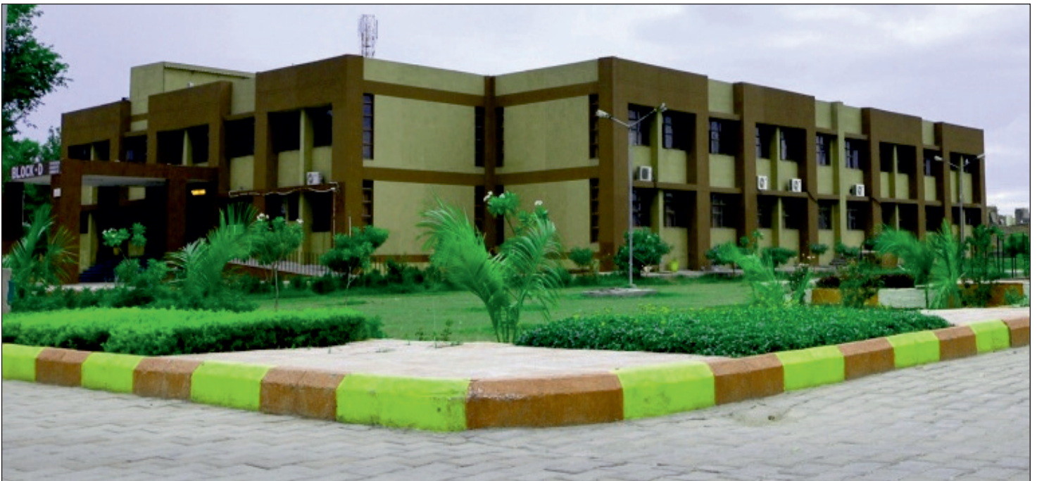
New Building Block-D that accommodates Administrative Sections and Polytechnic Wing
